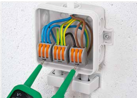
Testing the wired connectors
