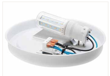
Connecting a light to the mains.
