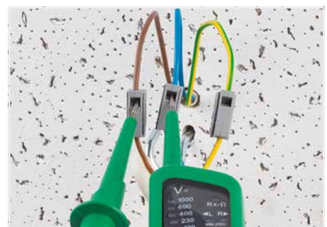
Testing via separate test ports.
